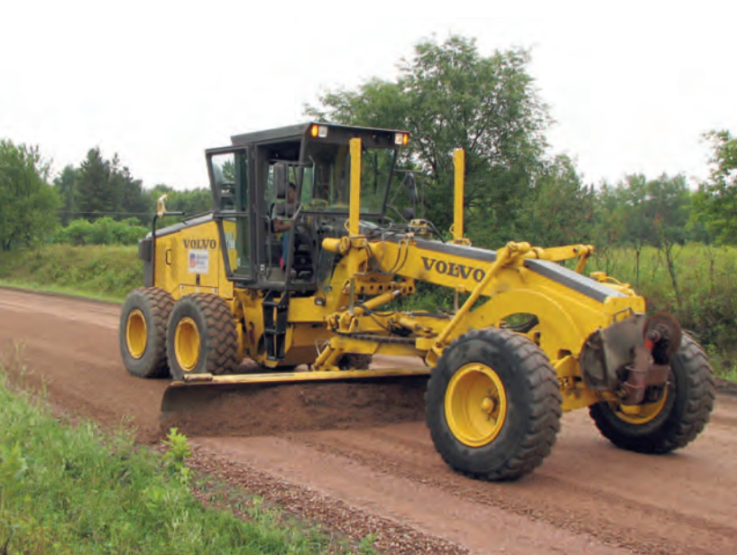
A worker prepares the road base for paving.
