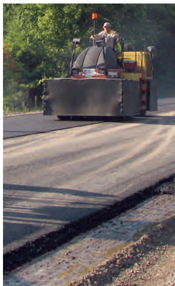
Applying final E10 asphalt layers.
