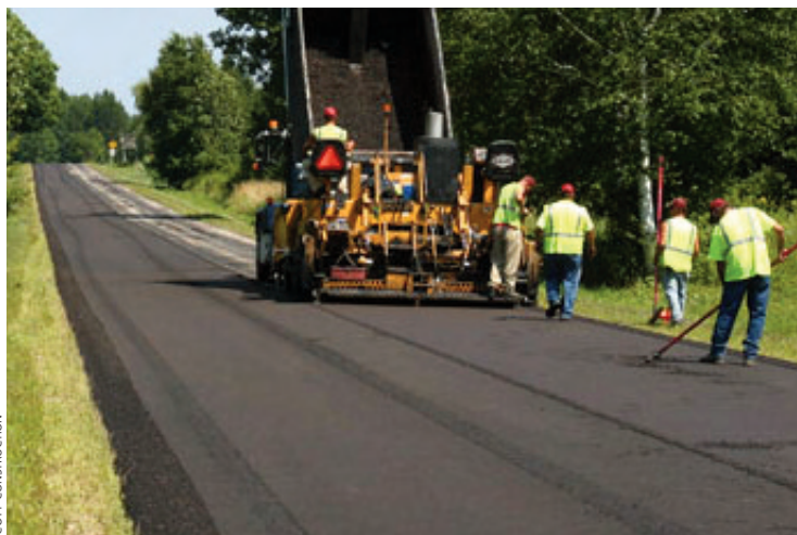
Cold mix paving on a town road in Sheboygan County.
