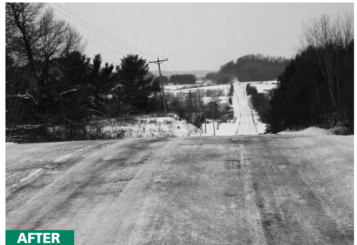
Looking west after realigning the road at the hillcrest and leveling the back slope.
