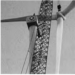
Crane hoisting turbine blades into position.
