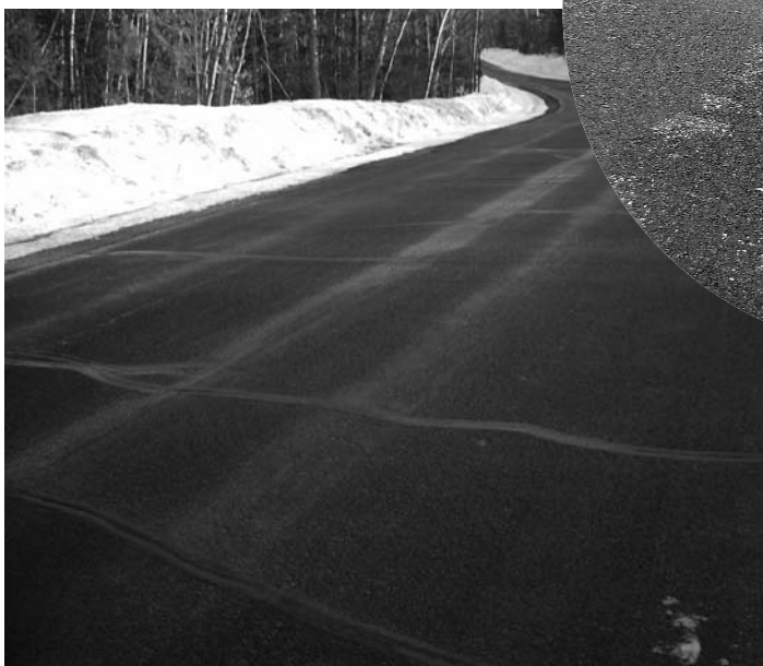
Sections of Gypsy Lake Road in the Town of Newbold pictured approximately eight months after application. Fog seal over new chip seal (upper left) and fog seal over existing chip seal (lower left). Close-up shows where the two tests meet with fog seal over existing surface on left in photo and applied over new chip seal on the right.
