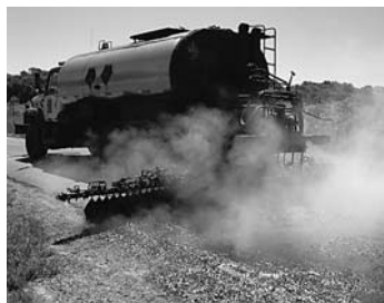
Work on a chip seal project.
