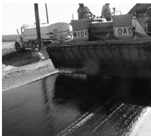
Streak caused by clogged nozzle.
