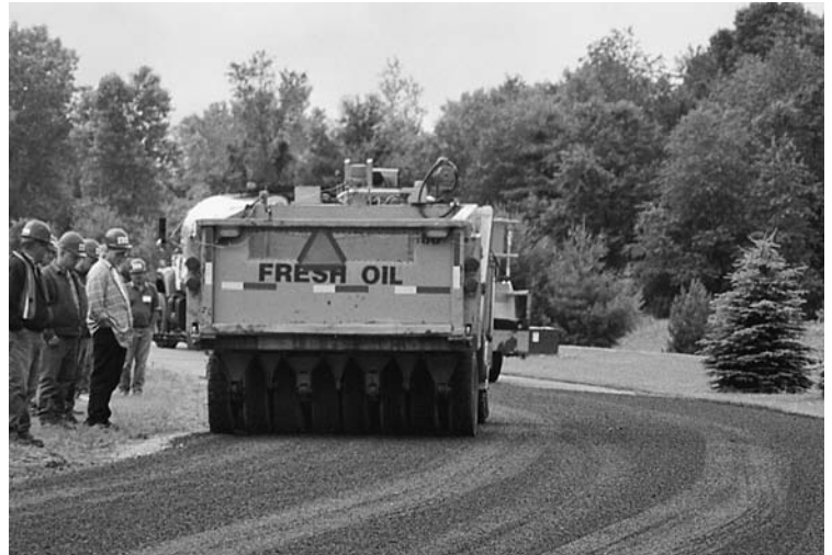
Rubber tire roller imbedding aggregate on a chip seal project.
