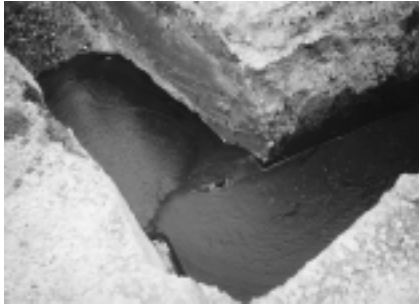
Asphalt fill flowing around corner of trench
