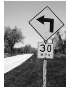
If the advisory speed is 30 MPH or less use a Turn sign.
