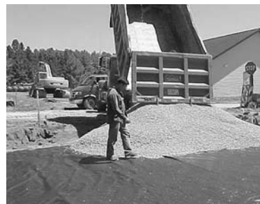
TOP: Careful installation of geotextile is important. БОТТОМ: Fabric holds clay back, keeping it out of the aggregate.
