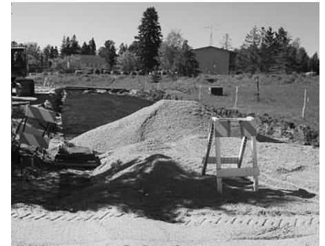
Using geotextile fabric over bad soils, like this clay on Madeleine Island, saves money and makes a better road.
