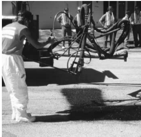
A – high pressure spray injection patching
