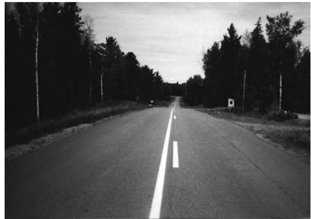
AFTER Slopes now meet modern design requirements. Utilities are moved, trees cut, and ditches built. To pay for these improvements, including purchase of more right-of-way, the Town of Bradley applied for and got a statewide TRIP discretionary grant from WisDOT and used part of the $500,000 it borrowed.
