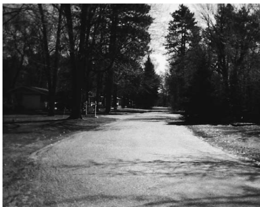
BEFORE This narrow (17 ft), urban road had no drainage and many trees needed to be removed.
