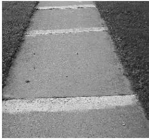
Sidewalk grinding
