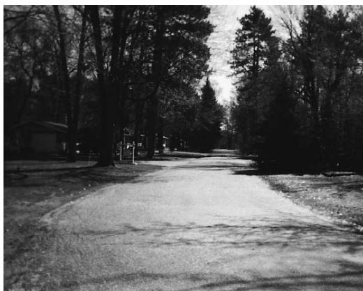
BEFORE This narrow (17 ft), urban road had no drainage and many trees needed to be removed.
