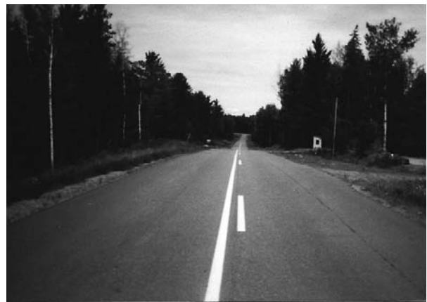
AFTER Slopes now meet modern design requirements. Utilities are moved, trees cut, and ditches built. To pay for these improvements, including purchase of more right-of-way, the Town of Bradley applied for and got a statewide TRIP discretionary grant from WisDOT and used part of the $500,000 it borrowed.
