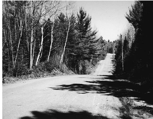
BEFORE Crass Road has many steep hills with very dangerous slopes, no drainage, and no place for snow removal.
