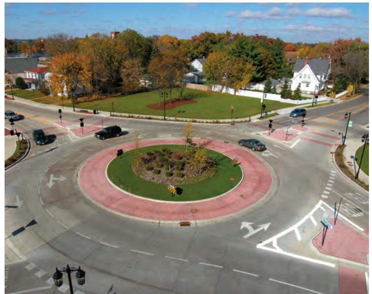
Roundabouts, like this one in Oconomowoc, are an intersection design gaining popularity in Wisconsin as a safety solution at certain locations.
