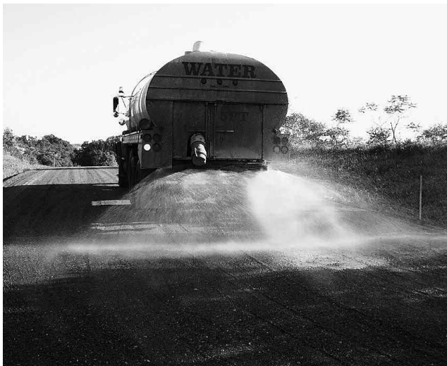
Jefferson County’s sprayer truck works road projects during the summer months, adding moisture to base materials.
