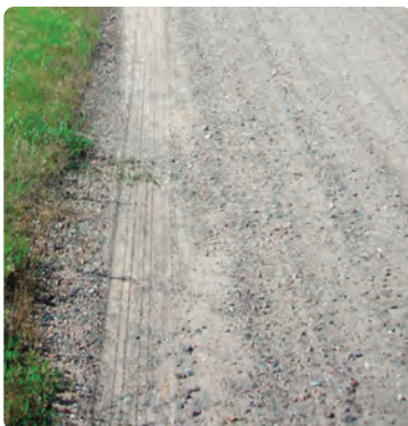
Controlling dust and stabilizing the surface means needing to grade a gravel road less often. Stabilization also keeps gravel fines bound in the road's surface.
