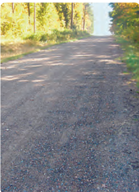
Sound design and regular maintenance keep gravel roads in good condition.
