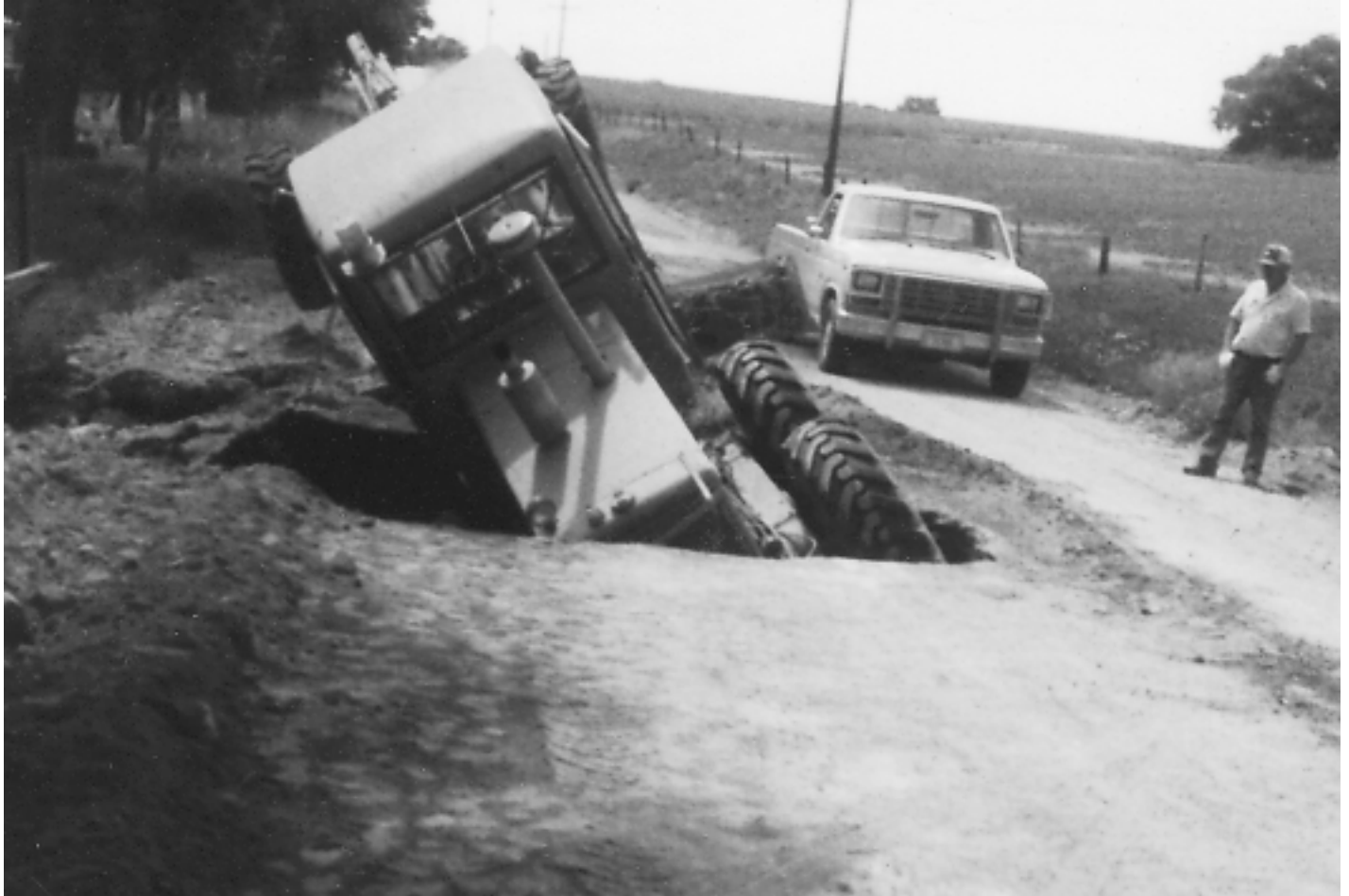
This road looked fine, but there was trouble brewing underground. Water travelling outside the culvert opened a six-foot high cave under the pavement that the soil had bridged until this last pass.
