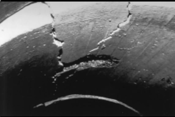
Poor support on the sides of this culvert allowed overhead loads to crack it.
