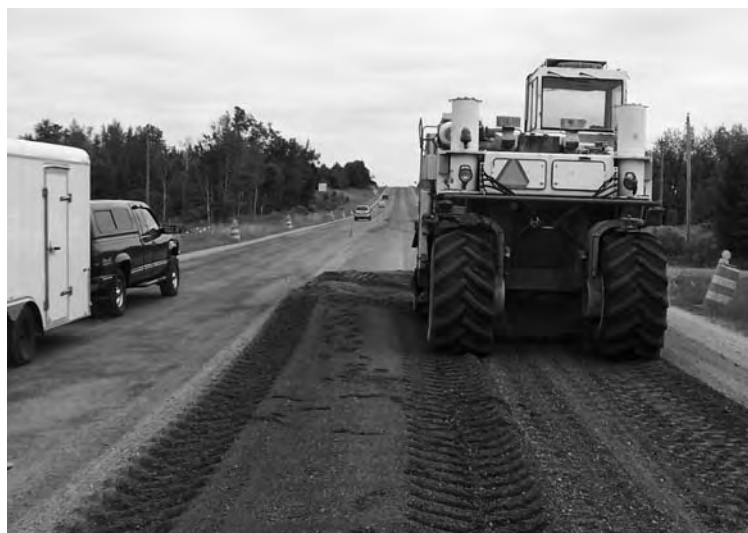
The pulverization process grinds and combines old asphalt layers with existing base materials to create a strong base for new overlay.
