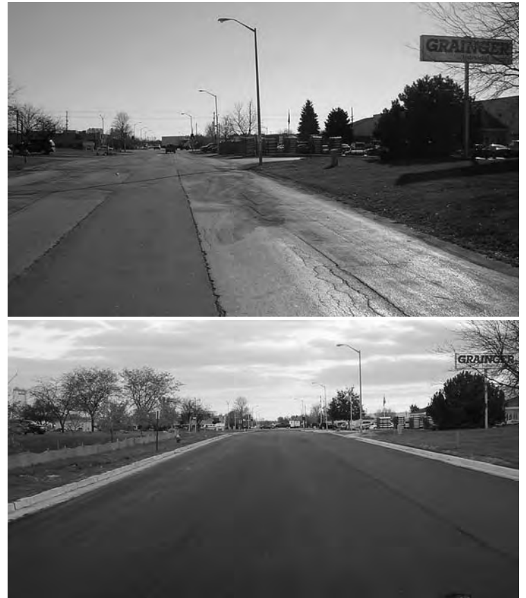
Before ABOVE and after photos of a section of the Northbranch Industrial Park road the City of Oak Creek rehabilitated in 2007 using pulverization. The project also added curb and gutter elements.
