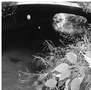
A healthy culvert.
