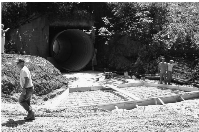
Culvert replacement work site.
