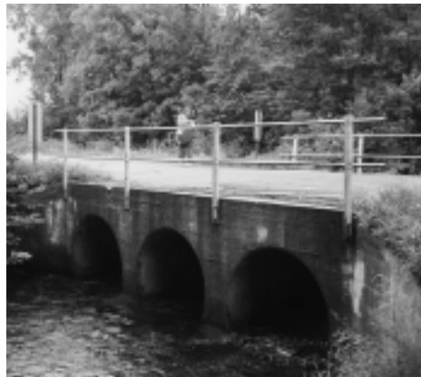
Bridge railing made of pipe is flimsy and dangerous (left). The intersection of County V and St. Patrick's Road is blind to drivers on both roads (right).
