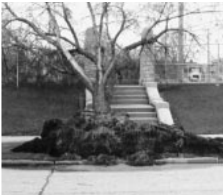
Construction practices killed this mature tree.
