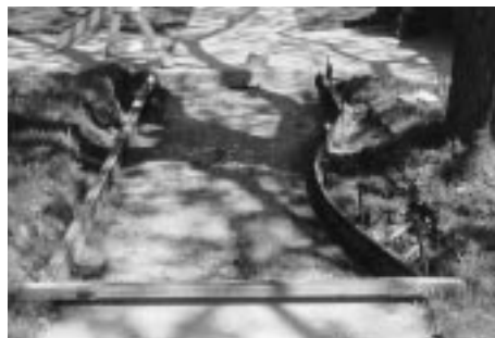
Protecting tree by arcing sidewalk.
