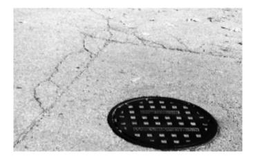
Pavement life goes down drastically around utility cuts—by five years according to a study in California; by seven to eight years according to a Vermont study. And, the best pavements suffer the greatest loss of useful life.
