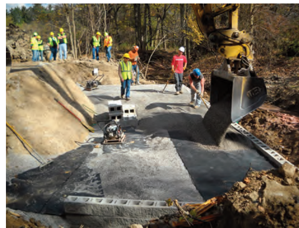
Photos taken by the FHWA's Joe Balice at a GRS-IBS project in Ohio show the process of preparing a foundation of compacted soil TOP LEFT , followed by placing layers of aggregate and geosynthetic fabric to the specified height of the structure, LEFT CENTER & BELOW . A wall of facing block, ABOVE , establishes the outer perimeter of the abutment.
