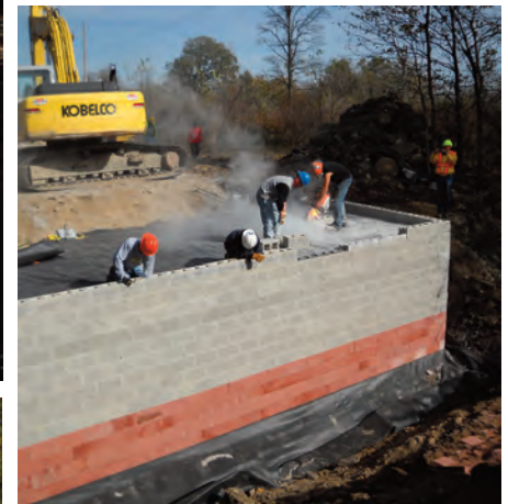
Photos taken by the FHWA's Joe Balice at a GRS-IBS project in Ohio show the process of preparing a foundation of compacted soil TOP LEFT , followed by placing layers of aggregate and geosynthetic fabric to the specified height of the structure, LEFT CENTER & BELOW . A wall of facing block, ABOVE , establishes the outer perimeter of the abutment.
